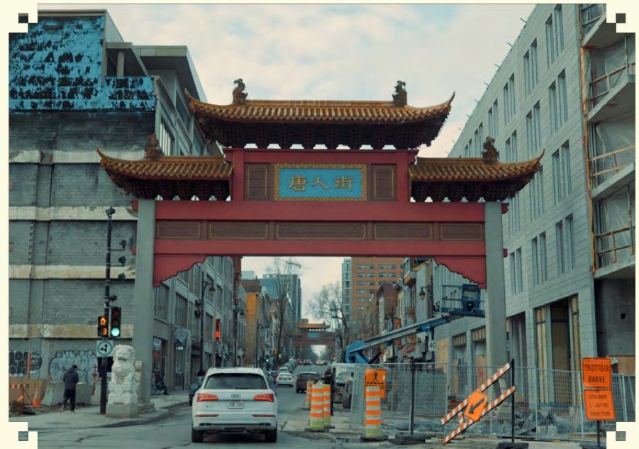
Montreal Chinatown Gate swallowed by condo construction Photo Credit: Van Royko
